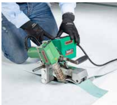
Thermal welding.
