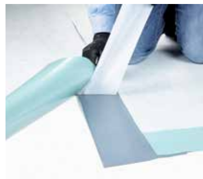
Sealing by butyl tape RENOLIT ALKORPRO BAND .
