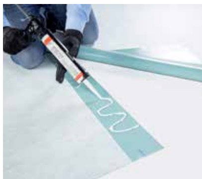
Sealing by mastic glue RENOLIT CEM 805 .
