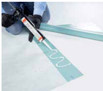
Sealing by mastic glue RENOLIT CEM 805 .
