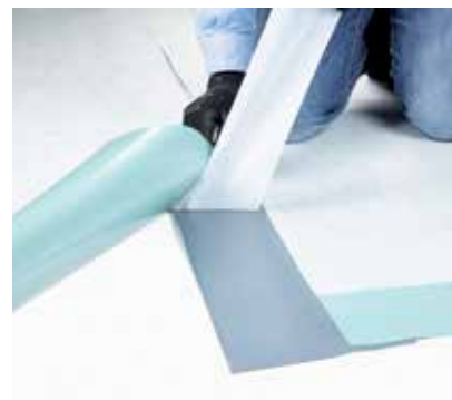
Sealing by butyl tape RENOLIT ALKORPRO BAND .
