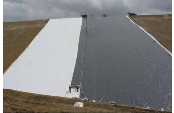
Unrolling and placing of geomembrane
