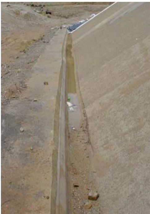
Principle of a flange construction to fix the lining system
