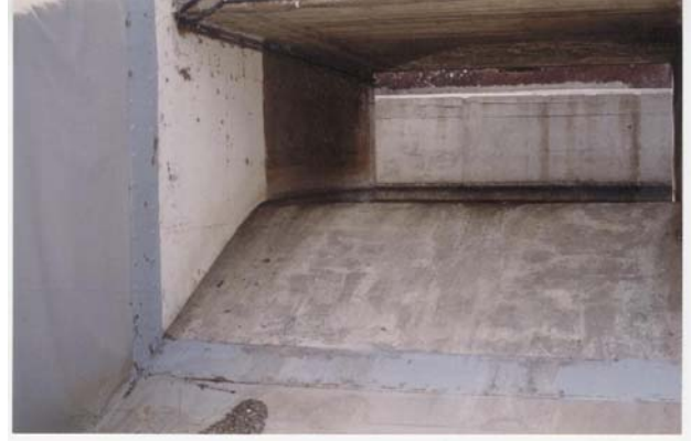
Connection to the concrete structure with the help of loose-fix flange
