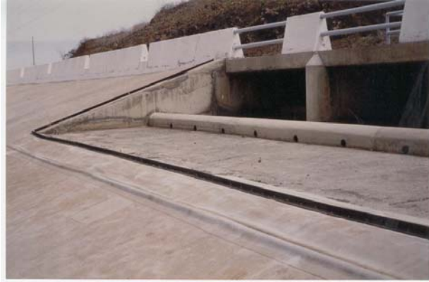
Connection to the concrete structure with the help of loose-fix flange
