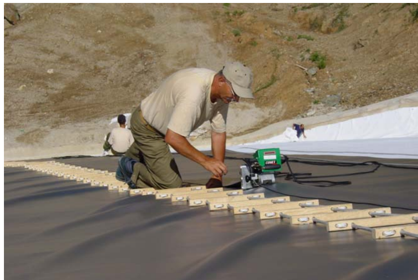
Welding with hot air and double seam
