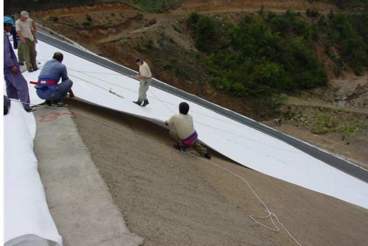
Placing of geotextile
