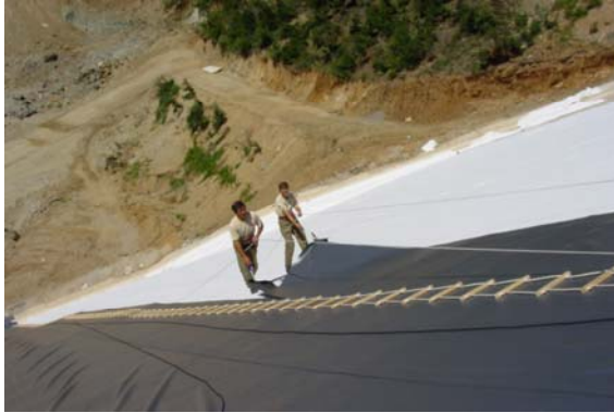
Unrolling and placing of geomembrane
