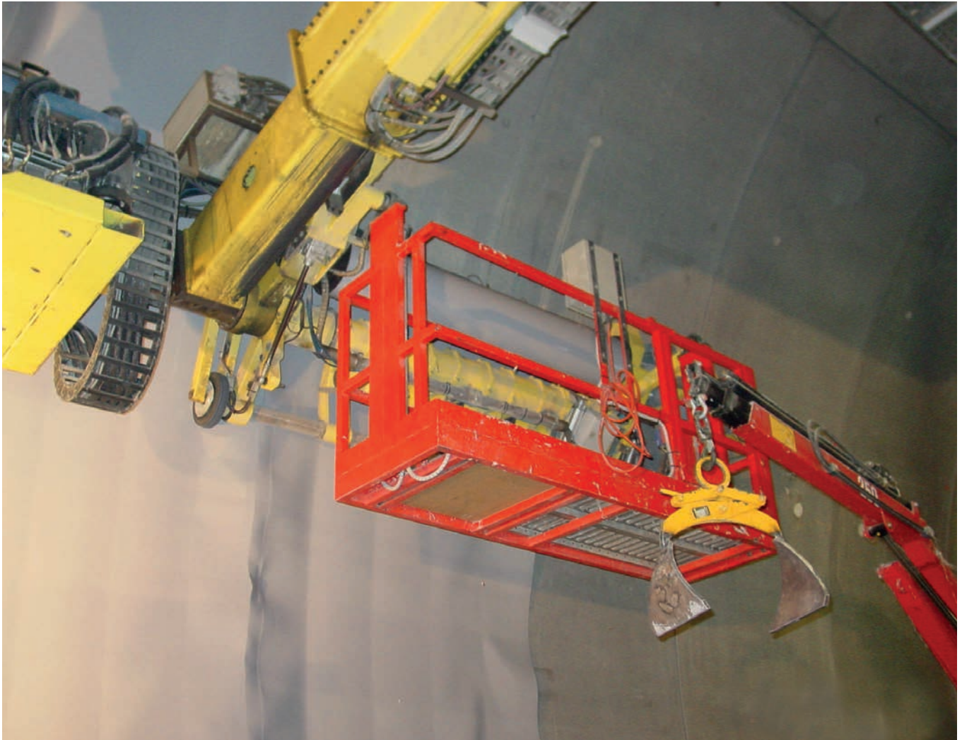
Installation geomembrane with glue
