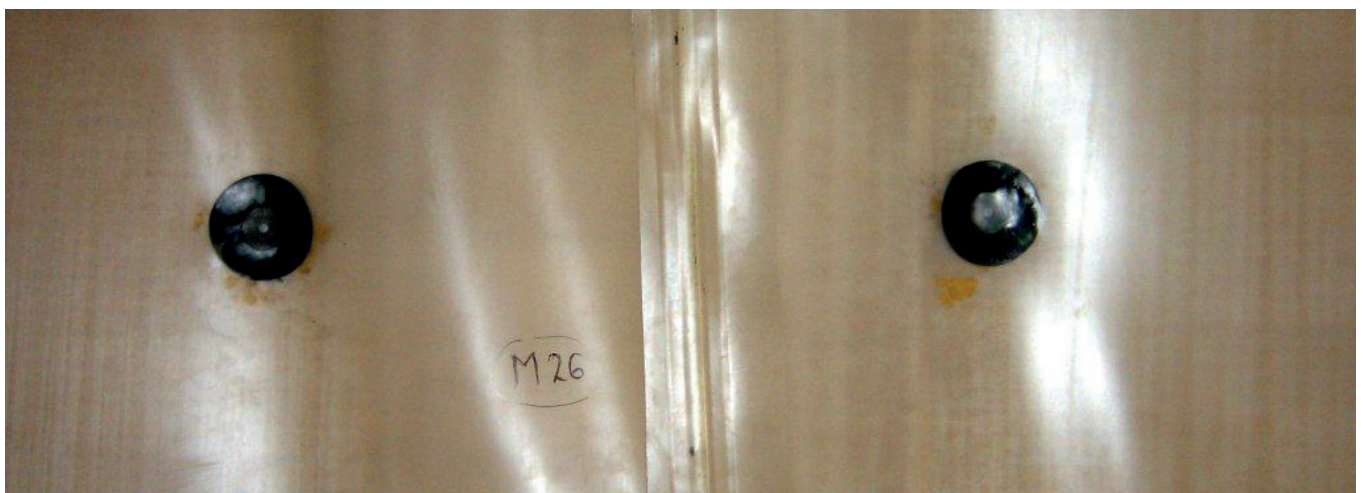
Fixation of the geomembrane by spot welding
