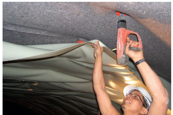
Fixation of the geotextile
