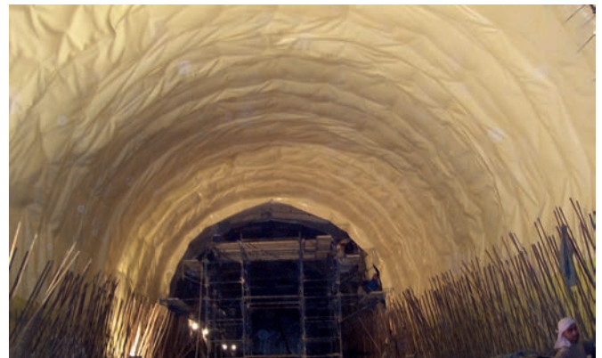
Scaffolding for manual installation
