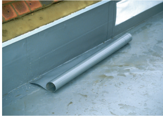
fig. 3: Edge restraint with RENOLIT ALKORPLAN 81170 or 81171 metalsheet
