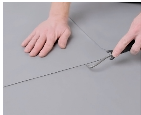
fig. 2: Verification of weld security
